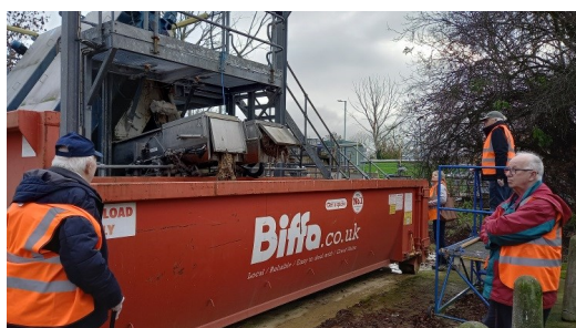
Rag—wet wipes, nappies, sanitary products ... the only ‘waste’ that goes to landfill
